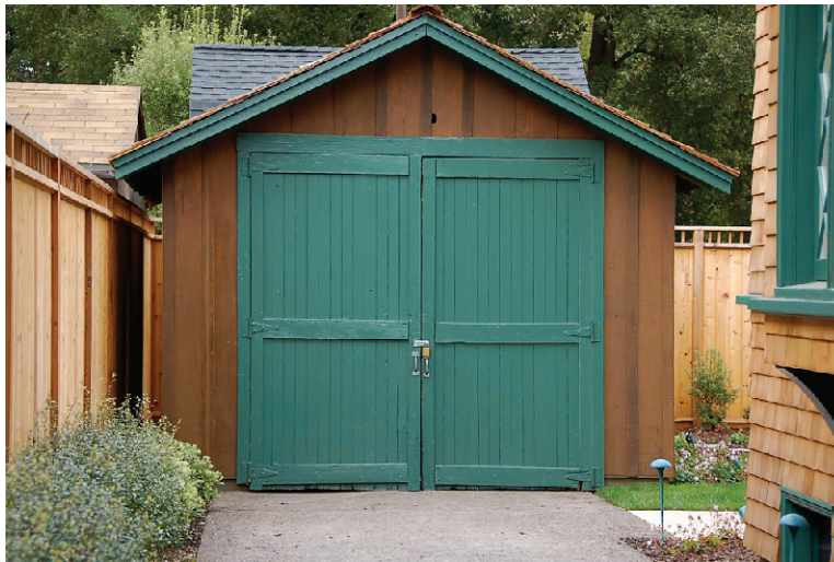
Figure 9.2 Hewlett-Packard has restored the original garage in Palo Alto, California, in which its two cofounders, Bill Hewlett and David Packard, former Stanford University classmates, began work in 1938 on the electrical switches and sound oscillators that became their new company’s first products. (credit: “HP Garage in Silicon Valley” by “MGA73bot2”/Wikimedia Commons, CC BY 2.0)
